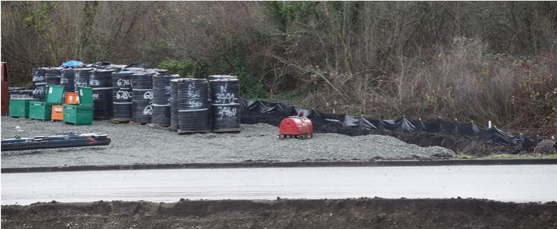
Plastic barriers are used to keep chemicals and debris from reaching Colquitz River during construction of the McKenzie interchange. But residents say mud and silt are spilling into the Colquitz River, threatening a coho spawning ground and a bird sanctuary. Photograph By ADRIAN LAM, TIMES COLONIST
