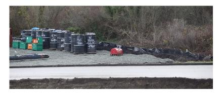
Plastic barriers are used to keep chemicals and debris from reaching Colquitz River during construction of the McKenzie interchange. Photograph By ADRIAN LAM, TIMES COLONIST
