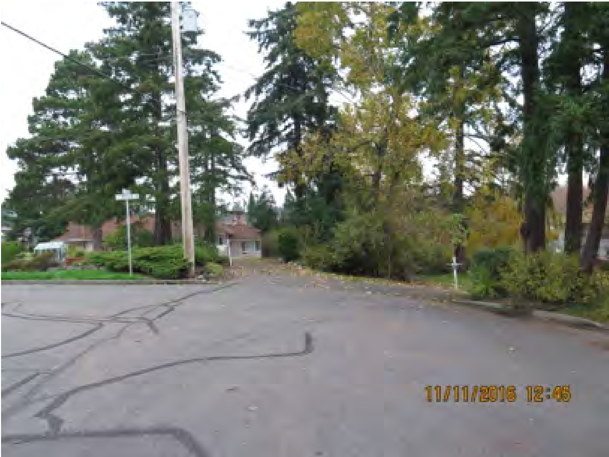
Figure 9.2 - Aral Road: facing North
