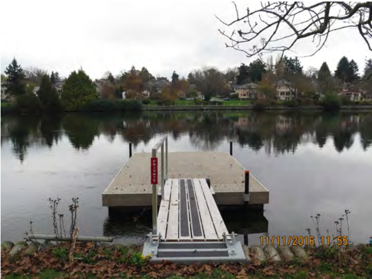
Figure 11.3 - Garthland Road: facing North
