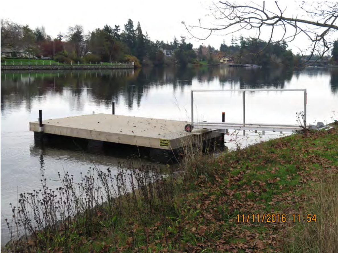
Figure 11.2 - Garthland Road: facing Northeast
