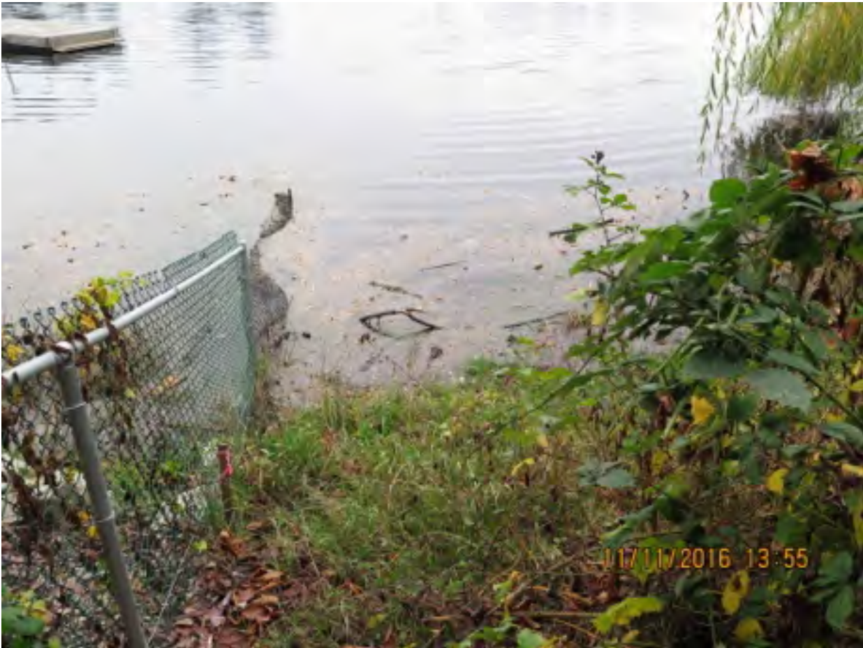
Figure 8.4 - Murray Drive: facing west from end of public access point
